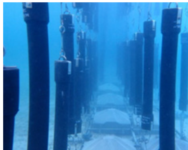
Sharksafe Barrier™ technology deployed at an island in the Bahamas. Credit: www.sharksafesolution.com
